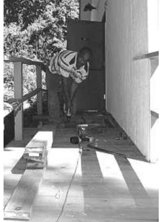
Sitiveni (Siti) Kete screwing on the deck boards
